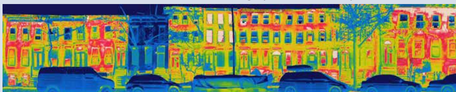
Figure 8. Thermal image showing external temperature of Tighthouse (fourth facade from left) and its adjoining neighbors.
