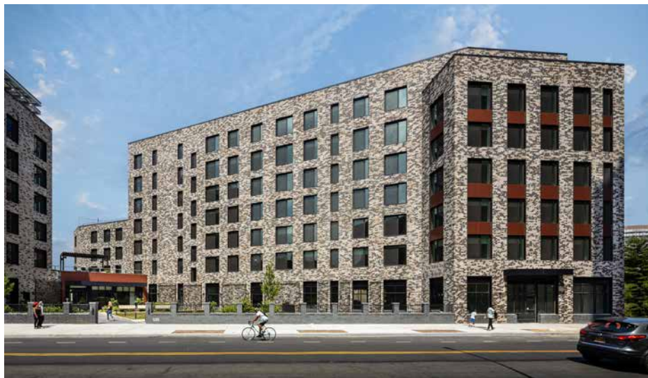
Figure 2. Vital Brookdale, a mixed-use Passive House building with structural steel at the ground floor and cellar, allowing flexible floorplate designs for its non-residential uses, and precast concrete planks and CMU bearing walls in the residential areas; the superstructures meet at the second-floor slab. The entry canopy is thermally broken structural steel, chosen to achieve the desired spans and cantilevered projection.
