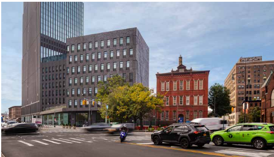
Figure 1. The mixed-use Alloy Block by Architecture Research Office includes New York City's first Passive House public schools: P.S. 456, the Elizabeth Jennings School for Bold Explorers, and the Khalil Gibran International Academy. The building's design strategy relates to two contrasting urban contexts: the major business and cultural thoroughfare of Flatbush Avenue for the high school entrance and the quiet, brownstone-lined State Street for the primary school. From mechanical dunnage posts to the tube-steel play enclosure, all structural elements that penetrated the insulation layer were equipped with polyurethane structural thermal breaks. Thermally broken brick shelf angles were utilized to maintain insulation continuity and avoid the linear thermal bridges typically found in brick-cavity wall construction.
