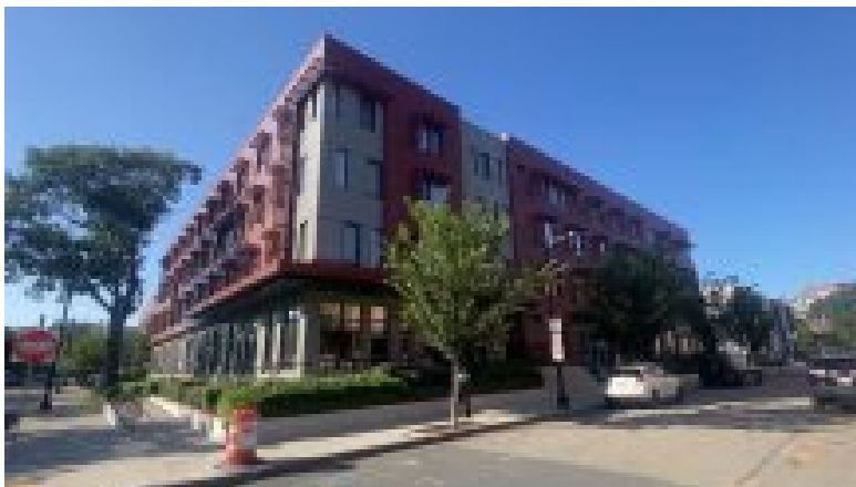
Senior housing at Anne Lynch Homes at Old Colony after the latest climate-friendly rebuild.
