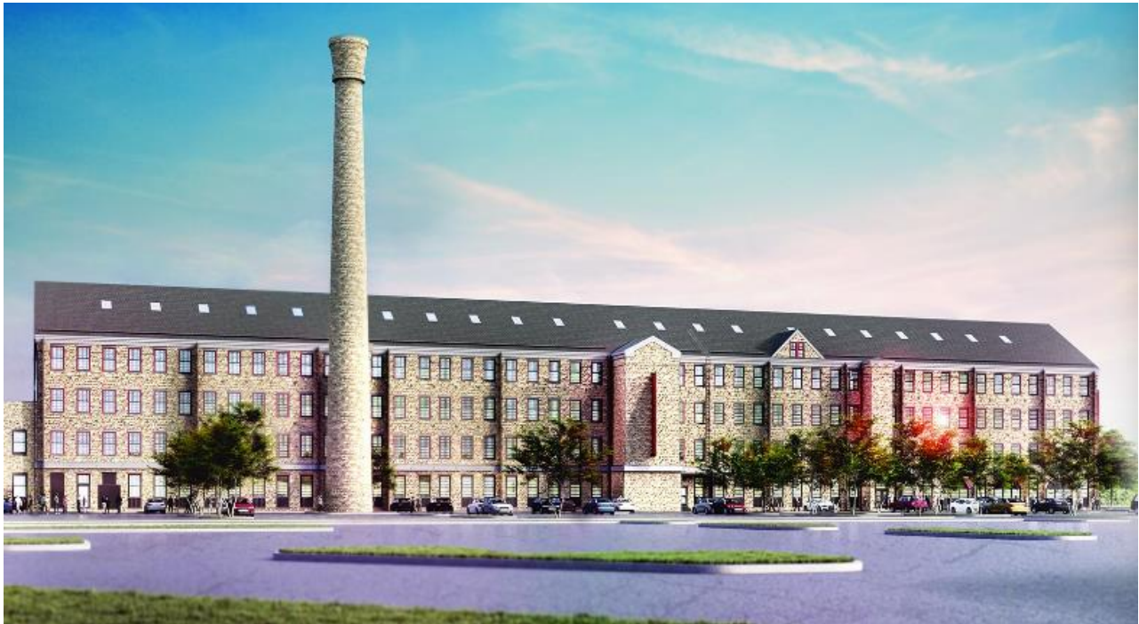
WinnDevelopment is redeveloping Lawrence's 177-year-old Stone Mill as an 86-unit mixed-income housing complex. Image courtesy of The Architectural Team
