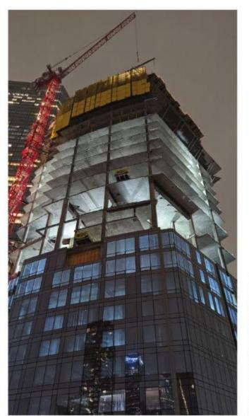
The construction process involved the simultaneous use of both creeper cranes and a tower crane, allowing the building team to enclose the tower on lower levels while forming and laying concrete slabs on upper levels.
