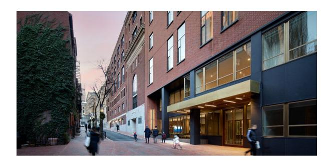
To create a cohesive internal transition between the two distinct six story structures, TAT stitched them together with a staircase and elevator banks, among other structural moves. The design team guided the restoration of the 1920s building's façade and reclad the 1960s modernist building with a new brick and granite skin. This approach forms a cohesive feel and shared architectural language for the two buildings, while preserving their architectural characters.
