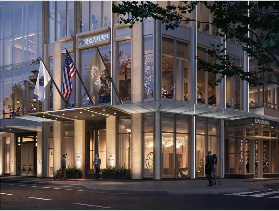
Credit: The Architectural Team // Binyan Studios
