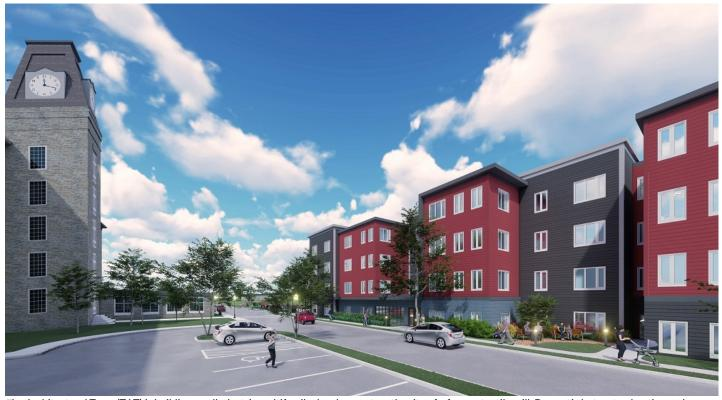
The Architectural Team (TAT) is building an all-electric multifamily development on the site of a former textile mill. Domestic hot water, heating and cooling are all electric. The four-story, 59-unit development is designed to consume zero net energy thanks to on-site renewables. Courtesy of The Architectural Team (TAT).
