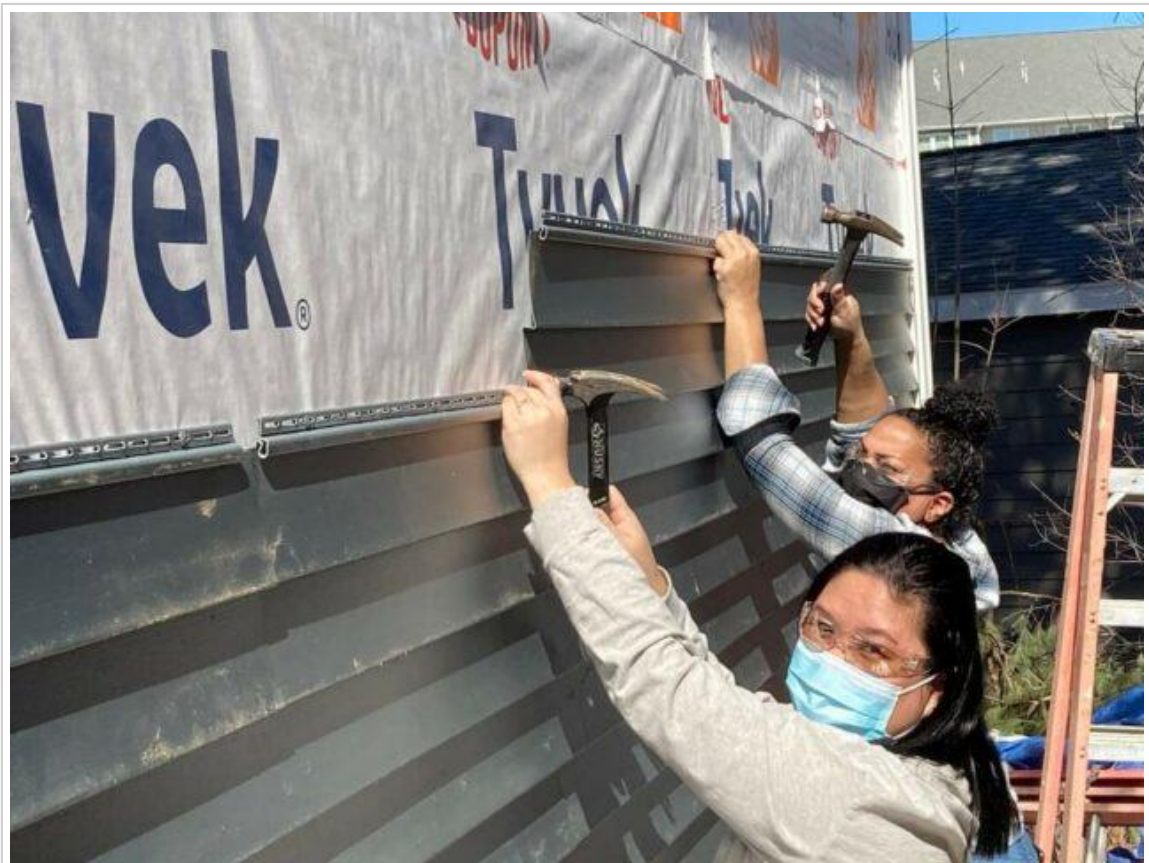
Littleton-based Workers Credit Union donated $5,000 to the Habitat for Humanity of Greater Lowell, and six employees volunteered to complete work on a house in North Billerica, including assistant vice presidents Chayanis Hauswirth (bottom) and Lissette Valdes. Photo courtesy of Workers Credit Union
