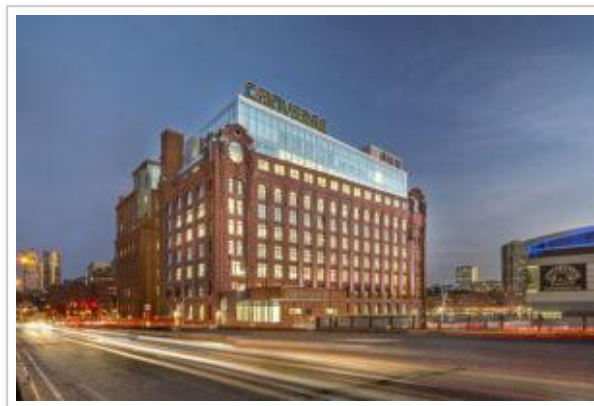
A modern glass addition to the Lovejoy Wharf property in Boston added square-footage while creating a bold waterfront statement. Photo courtesy of TAT
