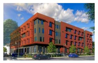
The Architectural Team's approach for the Anne M. Lynch Homes at Old Colony draws on staples of Passive House design, including robust, heavily insulated walls and high-performance windows, along with passive solar design and an emphasis on compact, simple geometries to reduce thermal bridges. A highly efficient HVAC split system further ensures a healthy and comfortable indoor environment for tenants. IMAGE: The Architectural Team
