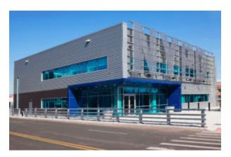
Spacesmith designed the LEED Silver-certified NYPD Auto Pound Operations Building, which is run by the Property Clerk Division. The design is clean and direct, utilizing an aluminum composite panel cladding system, low-e glazing and a PVC roof membrane. PHOTO: Tanya Braganti
