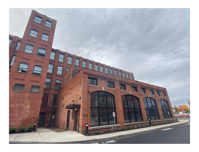
The building's existing masonry was repaired and the massive interior timber beams were retained. The large window openings were also preserved as approximately 1,300 new, high-performance, double-hung units from Diamond Windows & Doors were installed. The aluminum window frames were painted black to resemble old steel-framed factory windows from the early 20th century.
