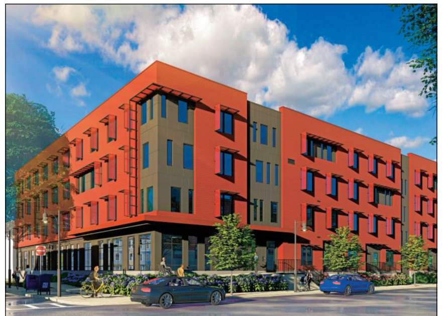
The third phase of redevelopment of the Anne M. Lynch Homes at Old Colony will include a 55-unit building for low-income seniors in South Boston.
