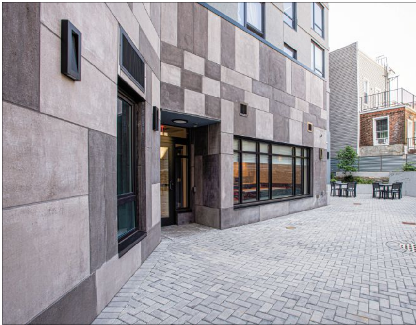
Home Street Residences rises eight stories on the former site of a vacant church in the Bronx, featuring 63 units of affordable housing for seniors.
