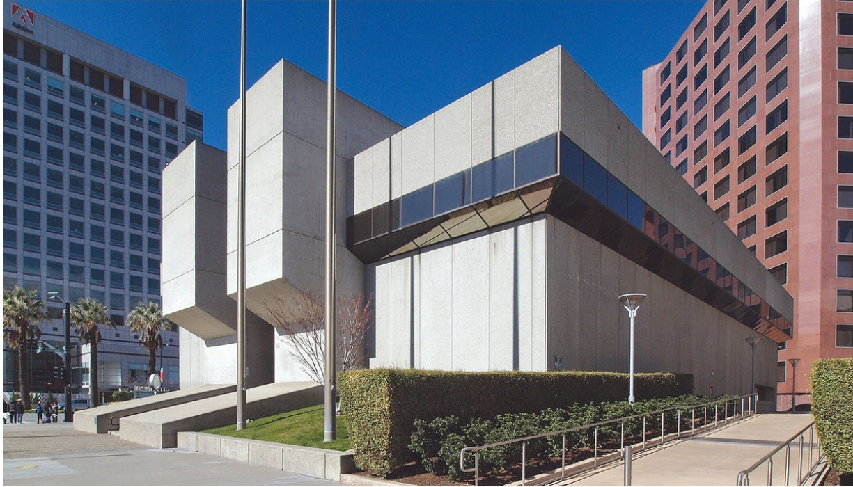
Bank of California Building in San Jose, California.
