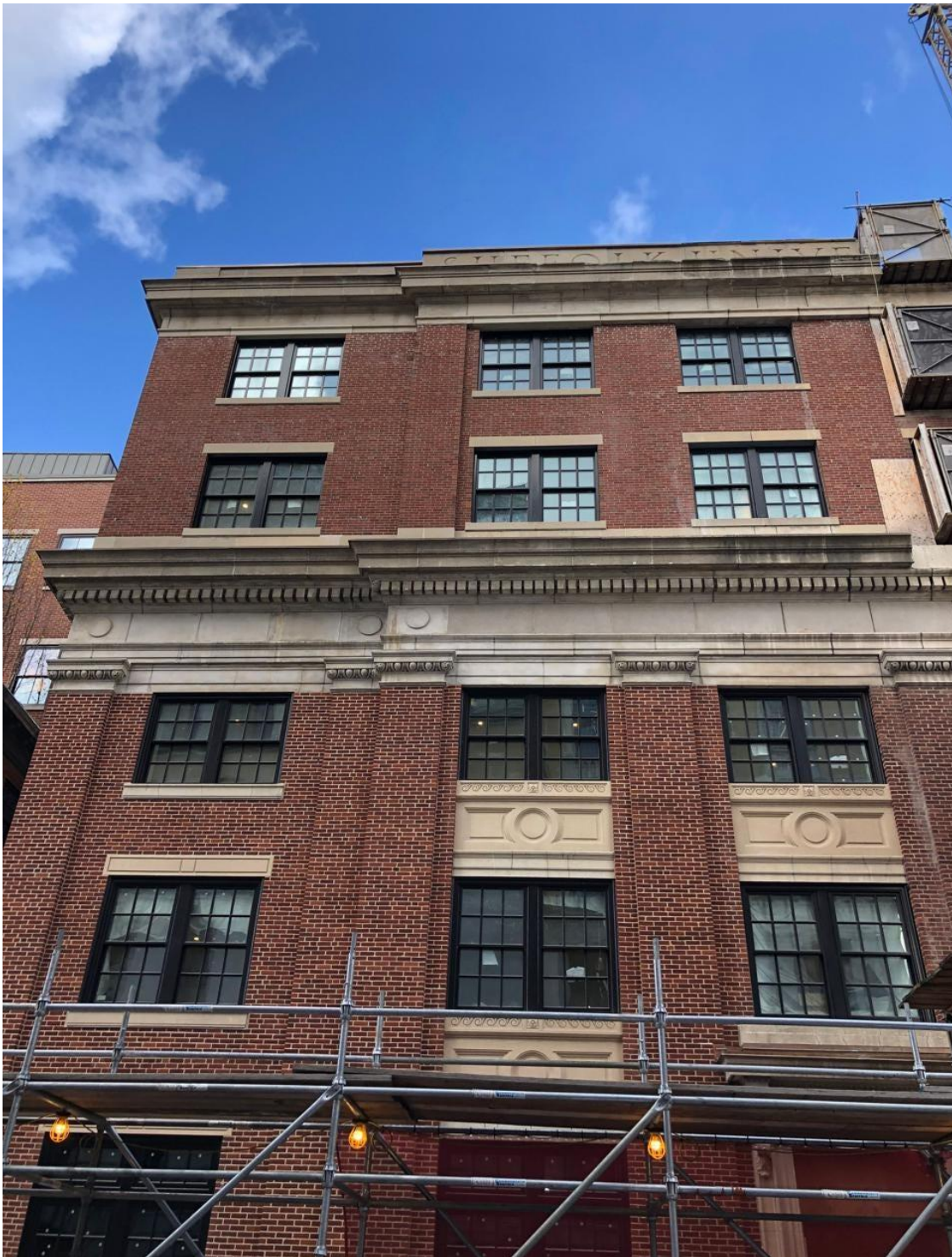
The exterior of the handsome 1920s building makes for interesting interior spaces. JARED KUZIA PHOTOGRAPHY
