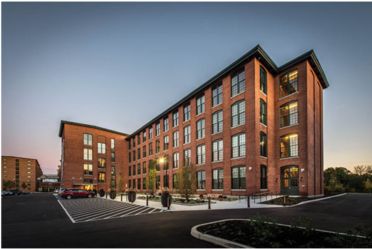
Built in 1907, Ludlow Mill 10, Ludlow, MA, remained derelict for nearly a decade prior to its rehabilitation and adaptation. The Architectural Team's work included a complete restoration of the structure and facade, as well as adapting the building's 108,000 sq. ft. to 75 modern apartments for seniors. Photo: Gregg Shuppe, courtesy The Architectural Team
