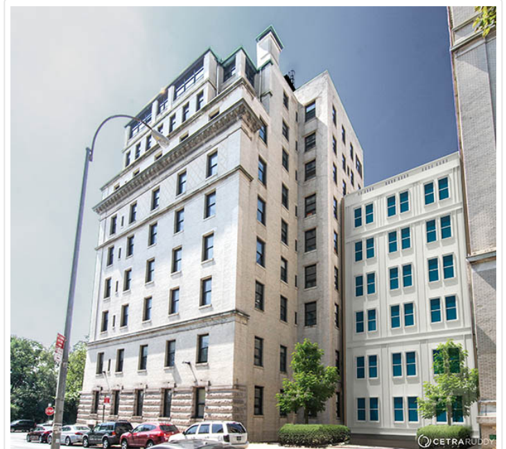
Located at 30 Morningside Drive in Manhattan, the residential conversion of the five Beaux-Arts structures formerly occupied by Mount Sinai St. Luke’s Hospital will retain the historic fabric of the existing structures in compliance with the historic landmark regulations, while also meeting all building code requirements.
