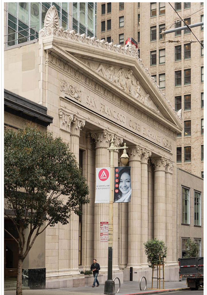
For the San Francisco Mining Exchange Building, Page and Turnbull used original terra cotta detailing to make casts for new terra cotta pieces, and made multiple in-person visits to ensure the replicas were sculpted and fired properly in the correct color. Photo courtesy Page and Turnbull.
