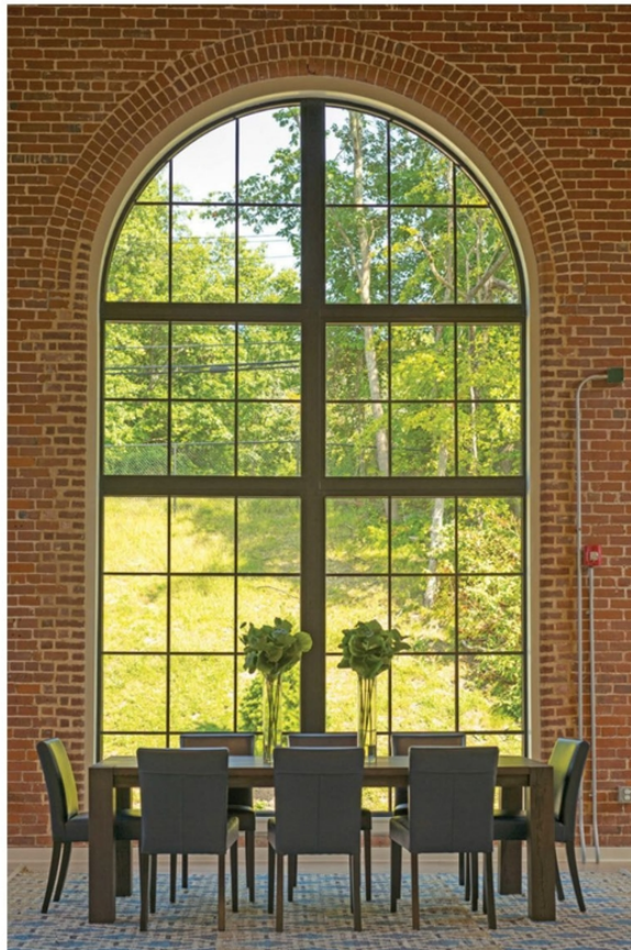
One of the building’s most notable features is its nearly 300 8-ft. x 10-ft. windows, which flood the interior with natural light. To meet NPS standards, the design team replaced original combinations of steel sash and wood frames with new, thermally broken aluminum frames featuring historically matched muntins and divided-lite windows. Photo: Andy Ryan, courtesy TAT
