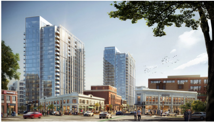
The Lincoln Common is a mixed-use development on the former site of Children's Memorial Hospital in Chicago's Lincoln Park Neighborhood consists of 1.1 million square feet, approximately 540 residential units, 105,000 sf of retail, and 68,000 sf of open space. Photo courtesy of Skidmore, Owings & Merrill LLP
