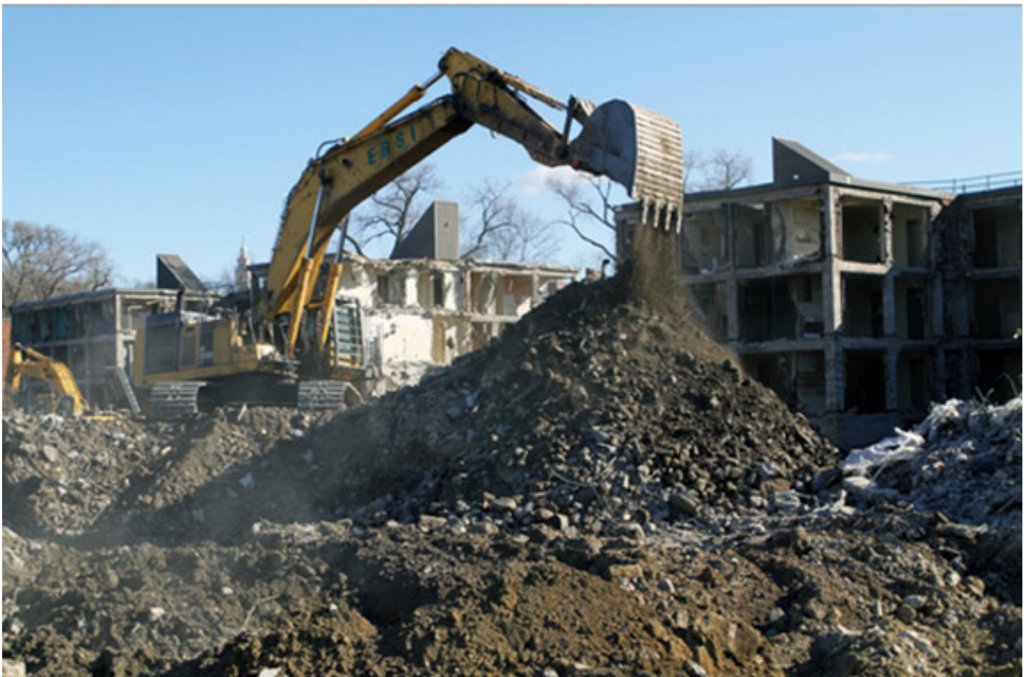
Bulldozers working at the Old Colony site Wednesday morning.
