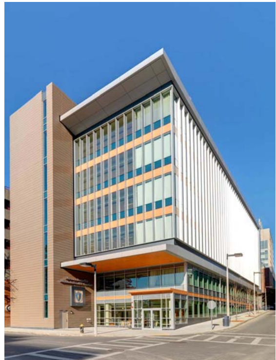
Clad with terra-cotta panels and curtain wall, the new Binney Street building is part of phase one. (Photo credit ©Andy Ryan)
