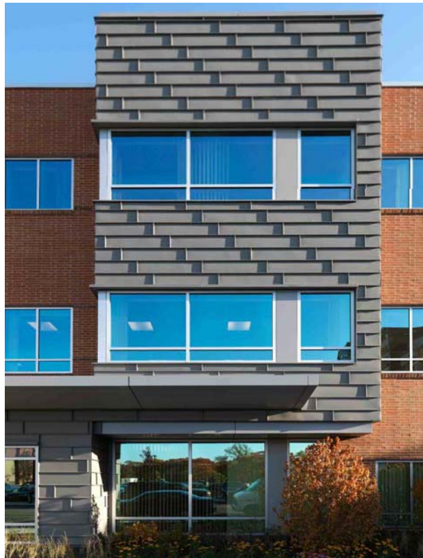
A new mental health day hospital, Fenwood Inn, opened in late 2011 as part of phase one of the redevelopment. (Photo credit ©Andy Ryan)
