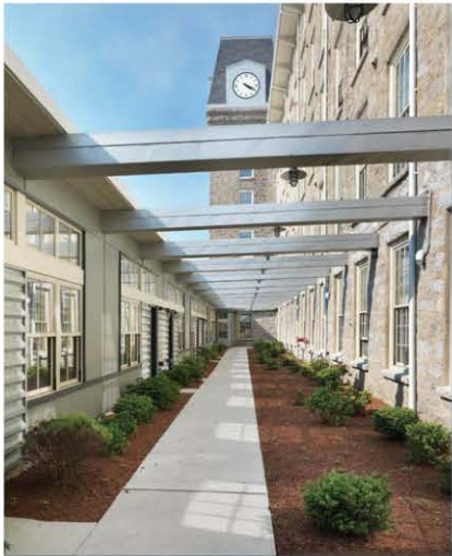
The Silver LEED Bourne Mill Apartments, Tiverton, RI, are the result of a project that converted eight mill buildings into a 165-unit residential complex. Many of the original features remain, including the locally quarried granite exteriors, the clock tower, and deep roof overhangs on the main building.
