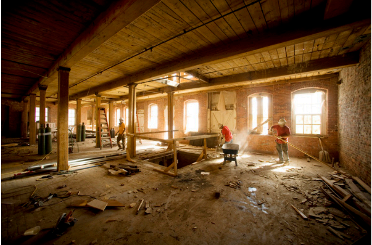
Early interior construction work. Photo credit: Greig Cranna, courtesy of MHP.
